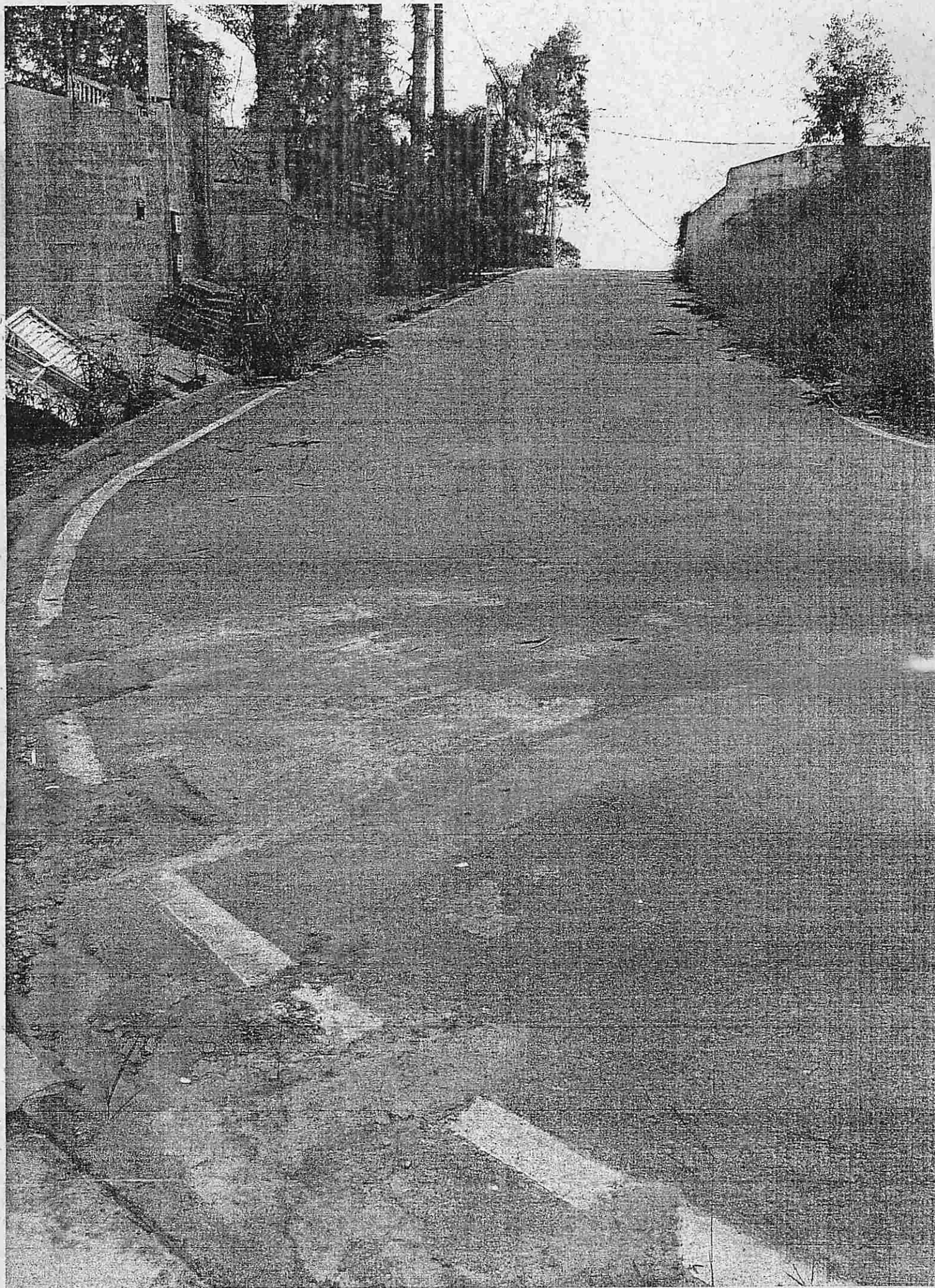
1) On the corner. Entrance to the On the mountain.
